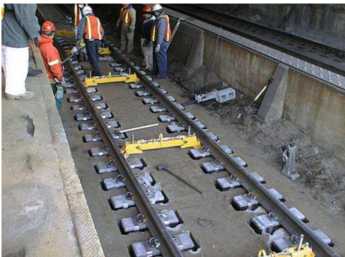
Track geometry re-adjustment
