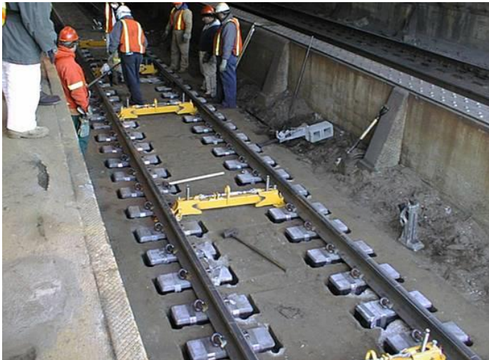
Track geometry re-adjustment
