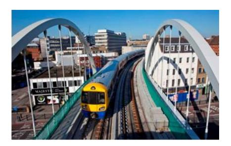
LVT Standard system with low tow fastenings was installed near the joint of the viaduct as observed in the photo below in order to allow the rail moves due to temperature gradients.
